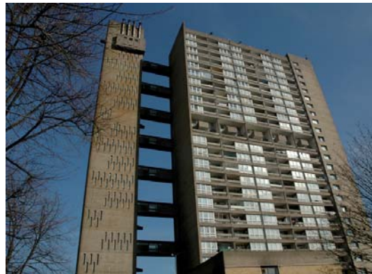
Balfron Tower, now part of the Bow Arts Trust live/work scheme
